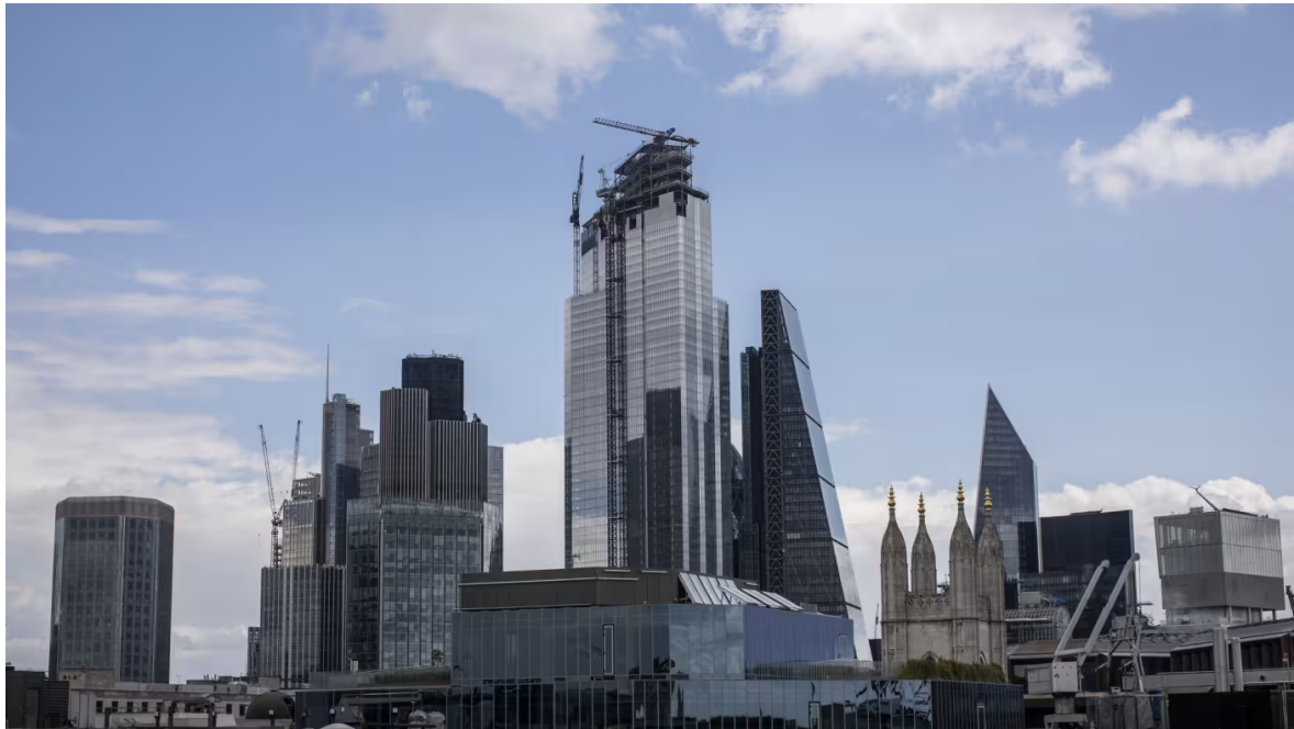
Construction is close to completion at 22 Bishopsgate, centre, in the City of London © Charlie Bibby/FT
