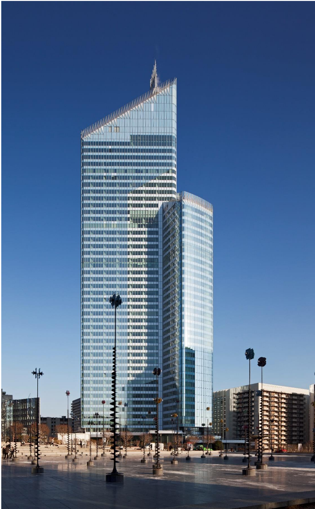
14/22 Tour First, La Défense, Paris, after renovation of the CB31 Tower. Karen Cook, while a partner at KPF, led the winning competition design to renovate the CB31 tower, for Altarea Cogedim and AXA into the Tour First. Jean Le Lay, while a Director at RFR, led the façade design. Source: Michel Denancé
