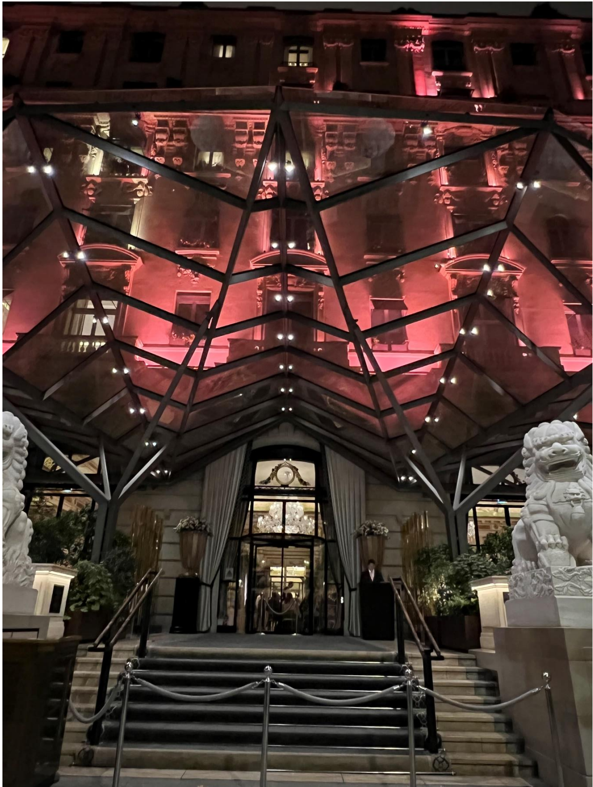
13/22 Hotel Peninsula, Paris. Design of steel and glass canopies led by Jean Le Lay while a Director at RFR Paris. Source: Mitsu Edwards
