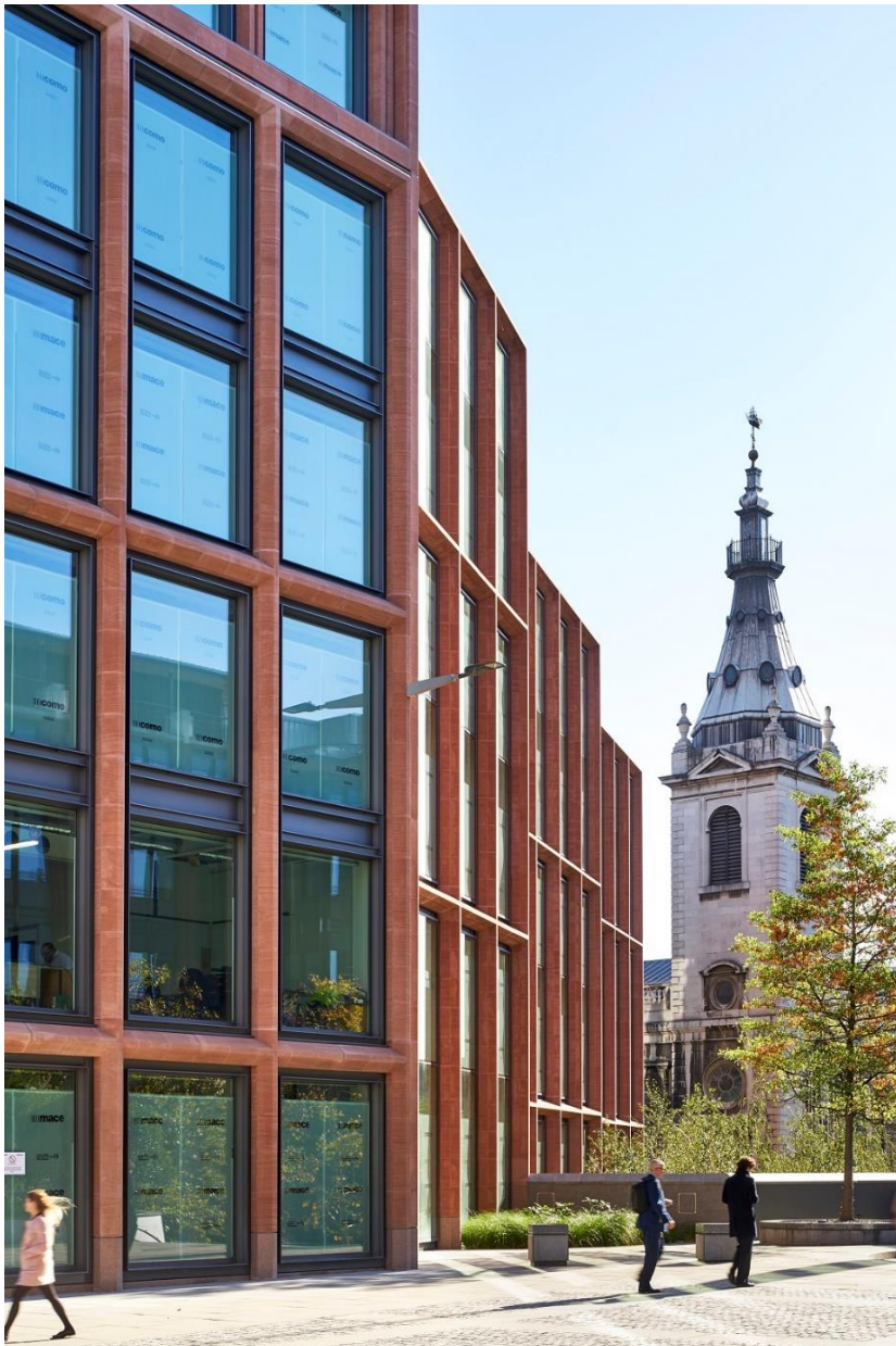
4 Cannon Street, City of London, steps away to reveal St. Nicholas Cole Abby. Design led by Karen Cook while a founding partner at PLP Architecture, for Pembroke on behalf of Fidelity. Source: Michel Denancé
