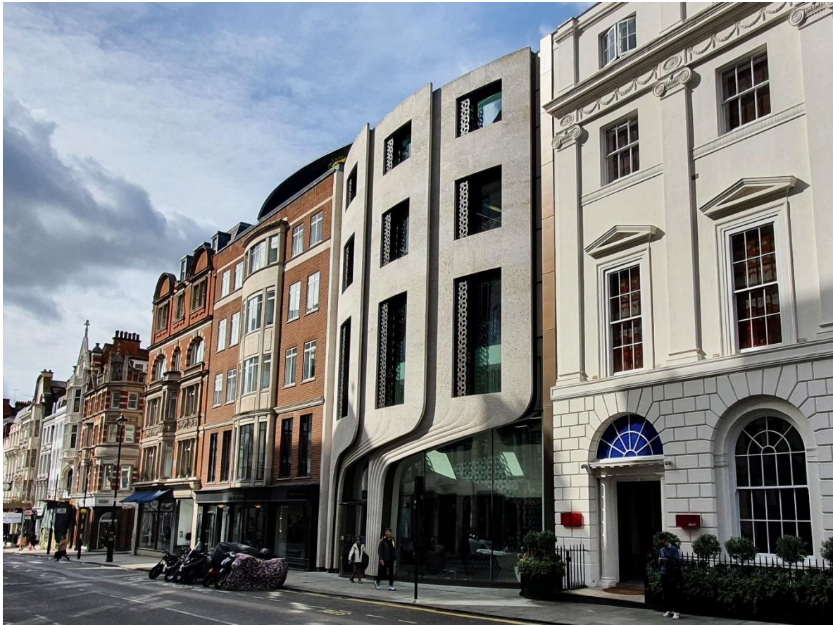
11/22 Qatar Airways London Headquarters, Conduit Street, Mayfair. Design led by Karen Cook while a Founding Partner at PLP Architecture, for Mace and Qatar Airways. Source: Karen Cook
