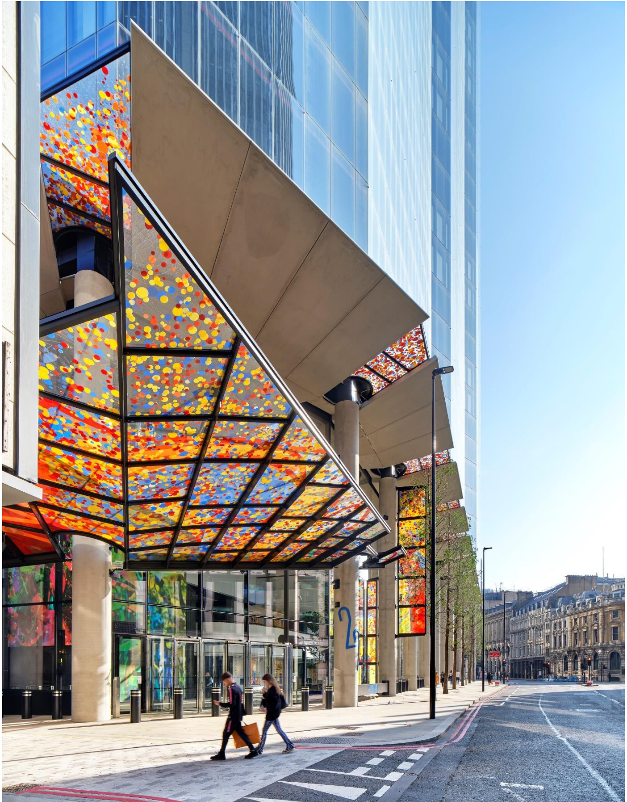
4/22 22 Bishopsgate north entrance. Canopy artwork by Alexander Beleschenko. Design led by Karen Cook while a Founding Partner at PLP Architecture, for Lipton Rogers and AXA IM. Source: Michel Denancé
