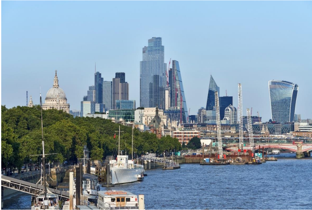
2/22 22 Bishopsgate on the City of London Skyline from Waterloo Bridge. Design led by Karen Cook while a Founding Partner at PLP Architecture, for Lipton Rogers and AXA IM. Source: Michel Denancé
