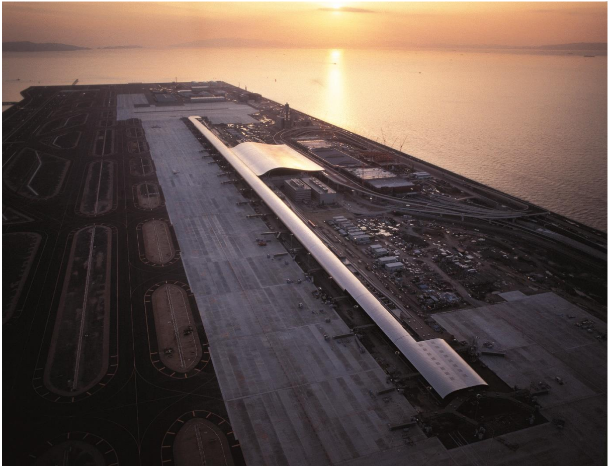
20/22 Kansai International Airport, Japan, architect Renzo Piano Building Workshop. Jean Le Lay was part of the winning design competition team while at RPBW Paris, moving to Genoa and then to Osaka to develop the design.
