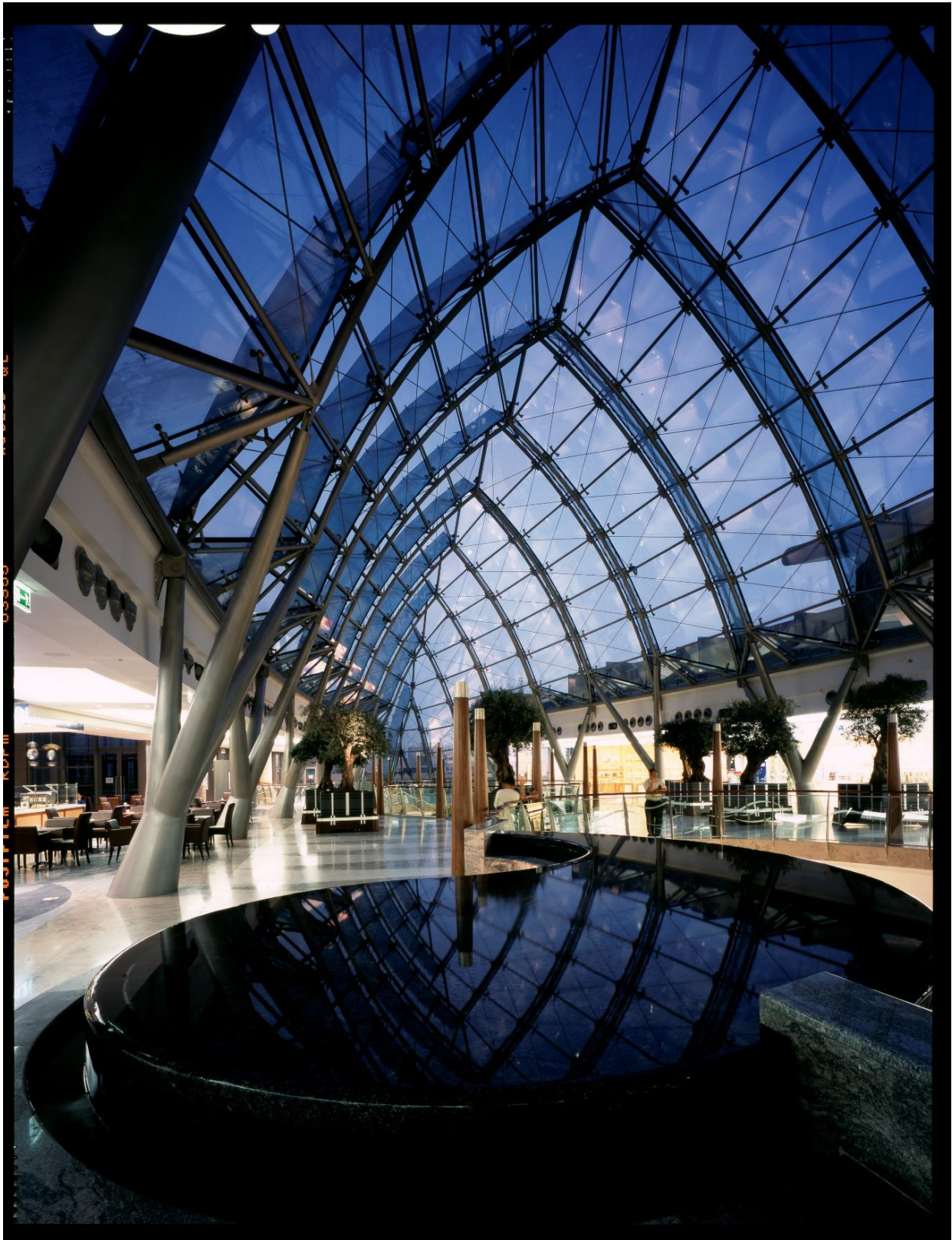
18/22 BurJuman Centre, renovation, Dubai. Interior view, South Village. Glass roof design led by Jean Le Lay while a Director at RFR Paris in collaboration with Eric Kuhne CivicArts and KPF London. Source: CivicArts
