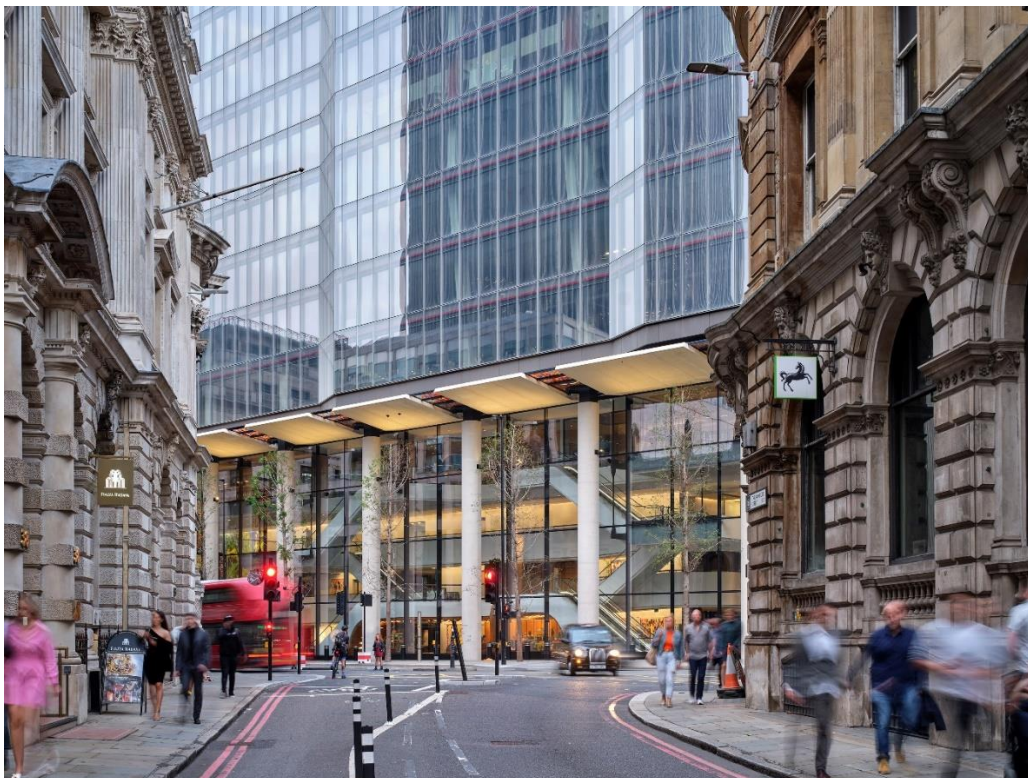
3/22 22 Bishopsgate from Threadneedle. Design led by Karen Cook while a Founding Partner at PLP Architecture, for Lipton Rogers and AXA IM. Jean Le Lay led the design concept of the canopy. Source: Michel Denancé
