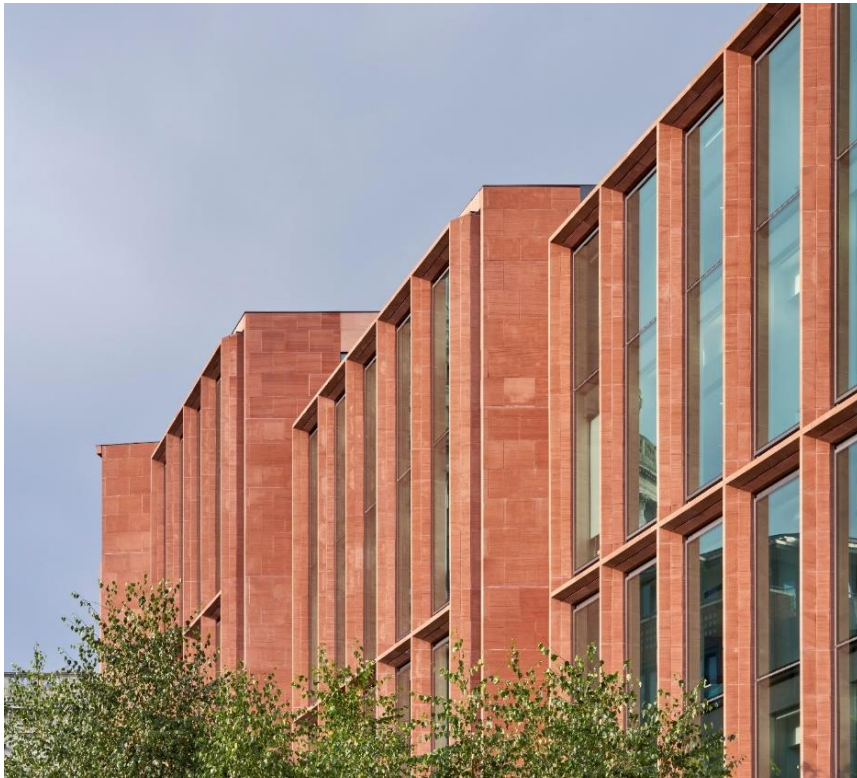
9/22 4 Cannon Street, southwest elevation, faced in Plimpton Red Lazonby. Design led by Karen Cook while a Founding Partner at PLP Architecture, for Pembroke on behalf of Fidelity. Source: Michel Denancé
